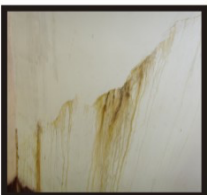
Seepage / leakage
